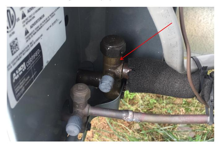
Large refrigerant pipe should be cool, similar to a cold glass of water. Cooling cycle should be running.
