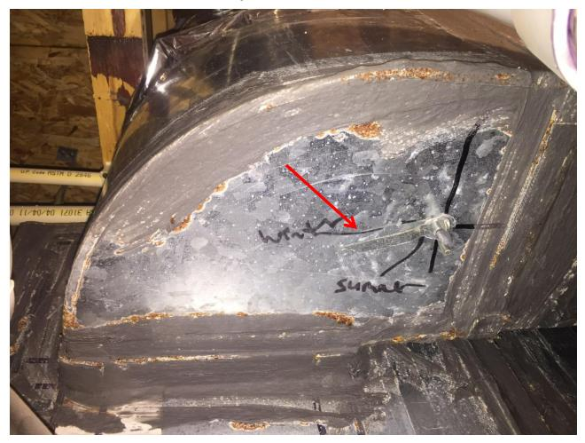
Restriction of airflow could convey to a furnace overheating. In case of a heat pump, it would raise pressure and can damage the compressor
